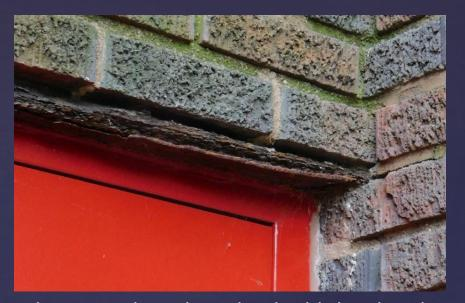
The original steel used to build the church is rusting and the rust scale is building up and causing damage to the adjacent masonry. In the above photo, the steel lintel located over an exterior door on the tower is severely rusted and bending the steel out of shape. In the photo to the right, steel embedded inside of the tower belfry has rusted and the rust scale has actually fractured the red clay tile block used to build the inner tower walls.
